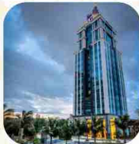
UB CITY, 15TH FLOOR VITTAL MALLYA ROAD
